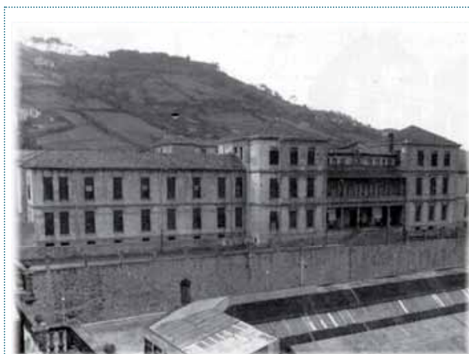
Hospital San Antonio Abad.
